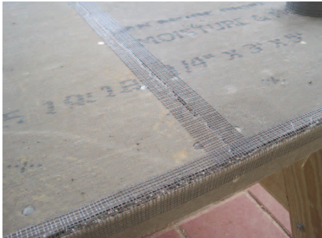
The seams where two different pieces of cement board touch should all be taped up with fiberglass mesh tape specifically designed for this job. The tape needs to be embedded in thinset mortar to function properly. The right photo is what it will look like when you are finished.
