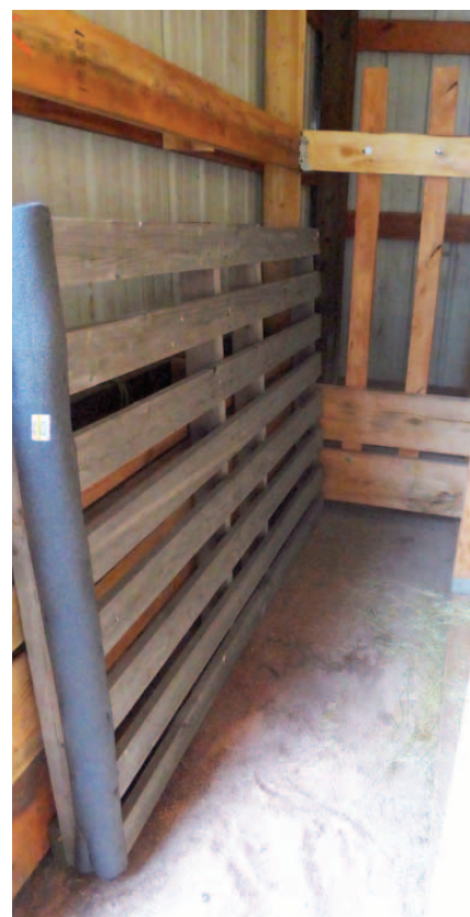
This is the pony wall forming the inside bumper of the milking stall (left). Because the milking stall ended up being too wide, we later inserted a 4x6 pallet (right) as a bumper in the milking stall; note pipe insulation on edge of pallet to protect Maggie from the sharp edge.
