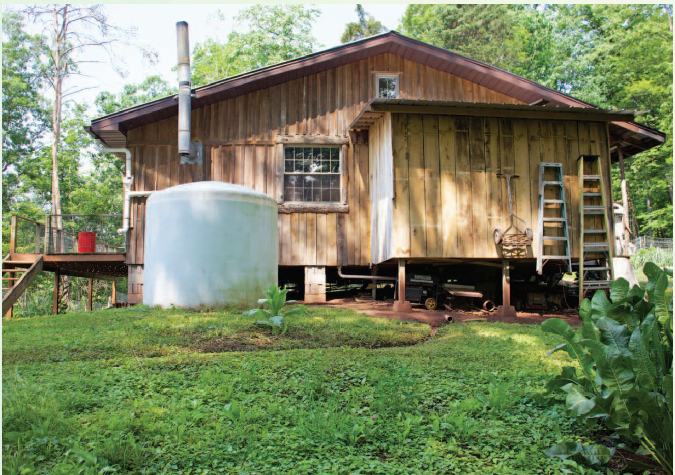
Our main water source is a 2,500-gallon tank fed by gutters off the roof of our 500-square-foot cabin.
