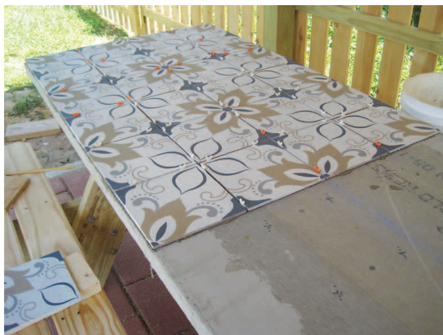
The tile is halfway finished.
