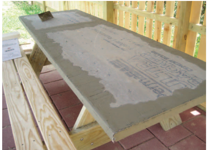
The seams where two different pieces of cement board touch should all be taped up with fiberglass mesh tape specifically designed for this job. The tape needs to be embedded in thinset mortar to function properly. The right photo is what it will look like when you are finished.
