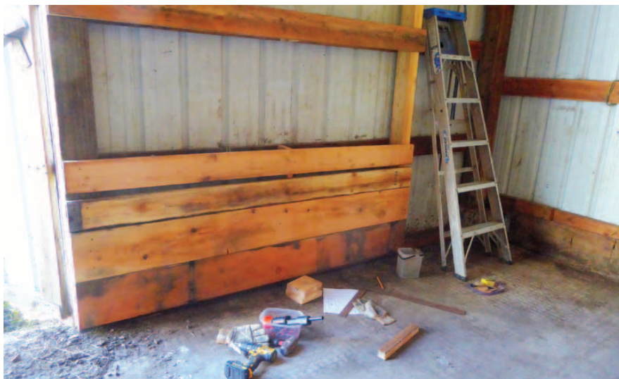
This is the pony wall forming the inside bumper of the milking stall (left). Because the milking stall ended up being too wide, we later inserted a 4x6 pallet (right) as a bumper in the milking stall; note pipe insulation on edge of pallet to protect Maggie from the sharp edge.
