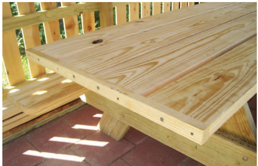
Here is what it looks like with the end piece of wood in place. Now the table is ready for the cement board.
