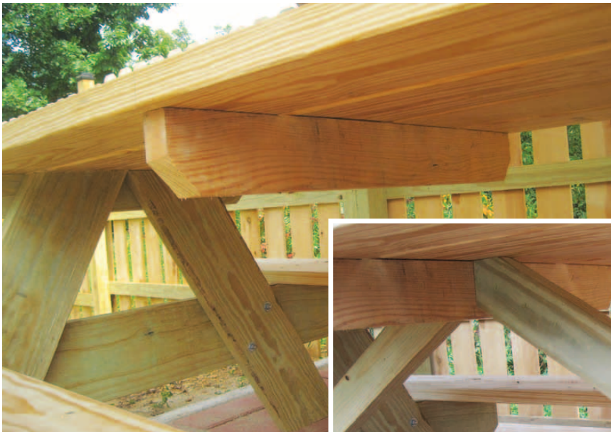
The picnic table top also requires a bit of extra support across the middle between the two frames. Attach the 2x4 as shown here. This support piece will also serve as a place to attach the diagonal support pieces. Right photo: Both diagonal supports are in place and fit snugly. Inset: Cutting one end of the diagonal support pieces in this manner helps them to fit better.
