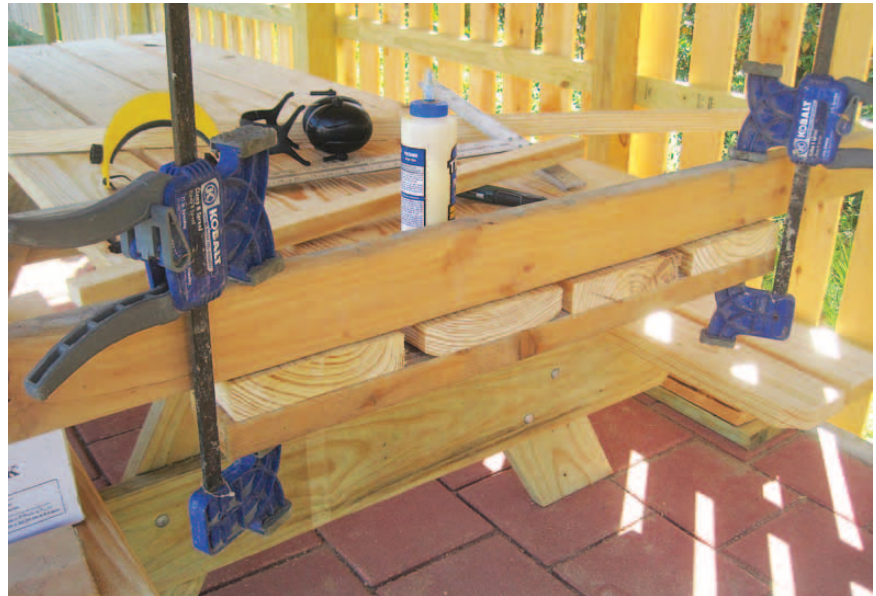
It is crucial that the end of the boards are perfectly in line before attaching the piece of wood to the end. Use clamps and scrap 2x4s to make this happen.
