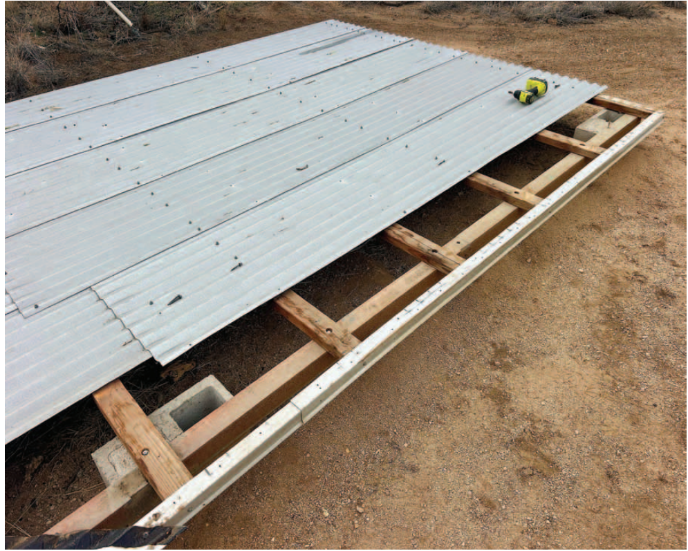
Rain roof is secured to purlin grid that sits on concrete blocks and metal stakes
