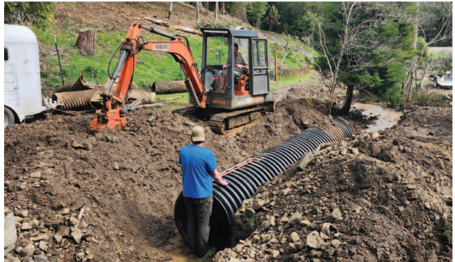
My sons installing a 40-inch culvert that we hope will be able to handle the debris if the creek floods again. The mangled smaller culvert is in the background.
