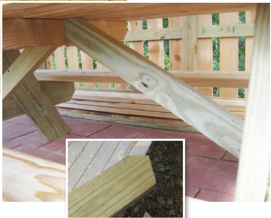
The picnic table top also requires a bit of extra support across the middle between the two frames. Attach the 2x4 as shown here. This support piece will also serve as a place to attach the diagonal support pieces. Right photo: Both diagonal supports are in place and fit snugly. Inset: Cutting one end of the diagonal support pieces in this manner helps them to fit better.
