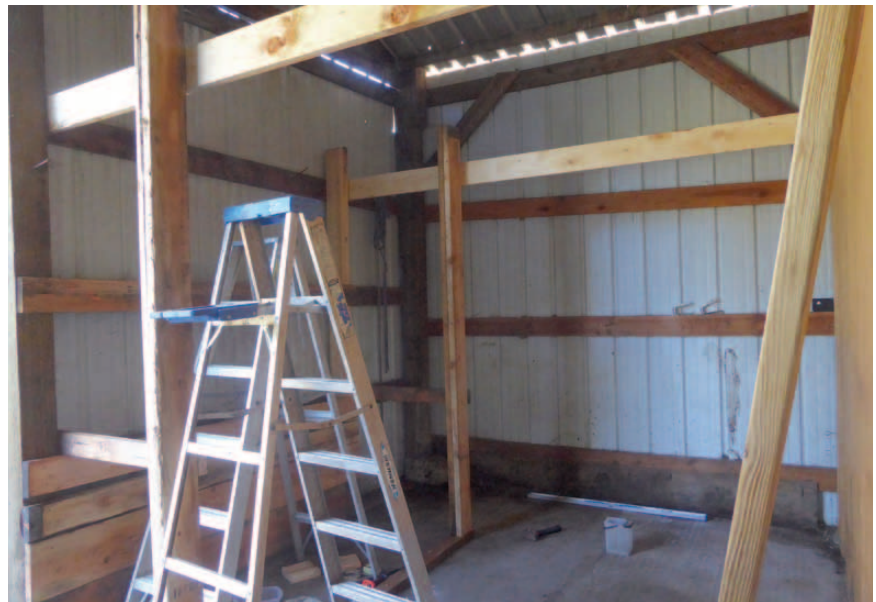
Upright posts tied overhead to 2x6 rafters for strength
