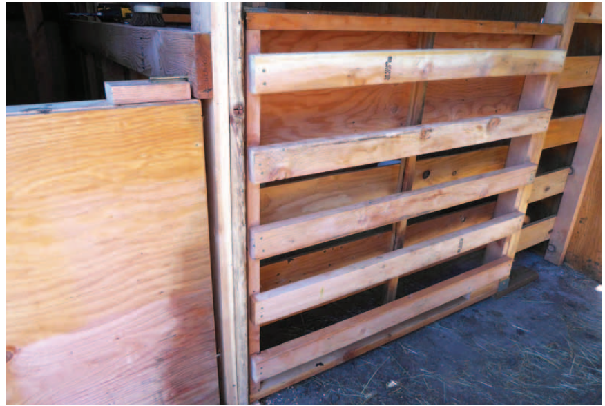
The outer milking pen gate is strengthened with 2x4 crosspieces.
