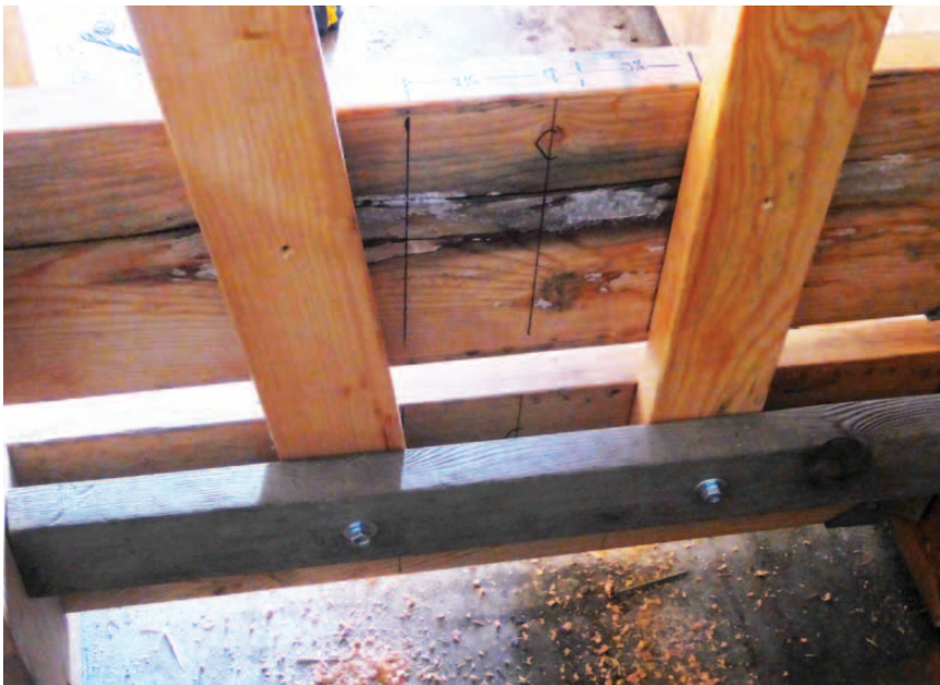
The base of head gate: 2x4s with bolts act as hinges so 2x4s can be moved and locked in place. The grain bucket is in the alcove on other side of head gate.
