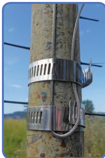
We threaded the steel cable through the eye bolts at the top of the pipes. Once the pipes were finished, we pulled the cable tight by hand, then affixed the cable to the pipe using hose clamps.
