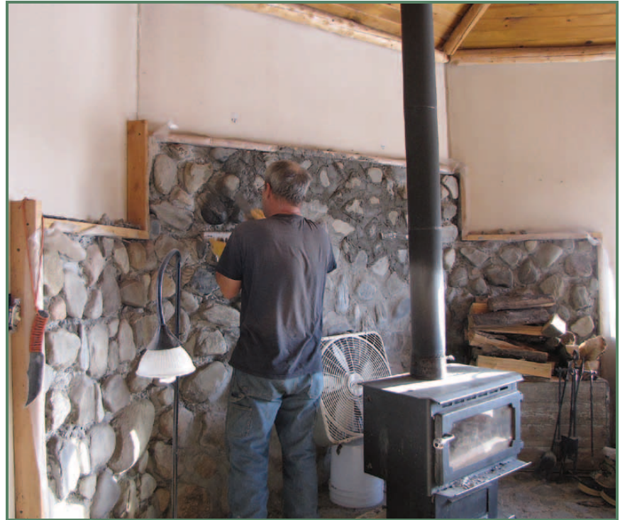
For safety and heat retention, Will built a stone hearth and surround wall for our woodstove in the living room.
