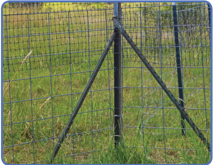
We used metal braces for added strength on the corner posts.
