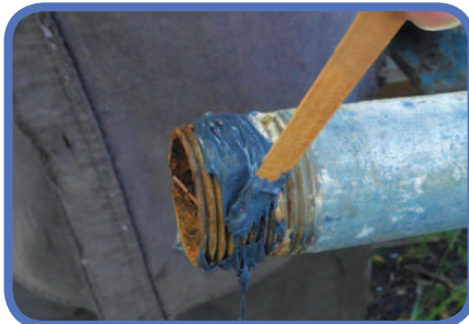
Using J-B Weld to affix an end cap to a pipe
