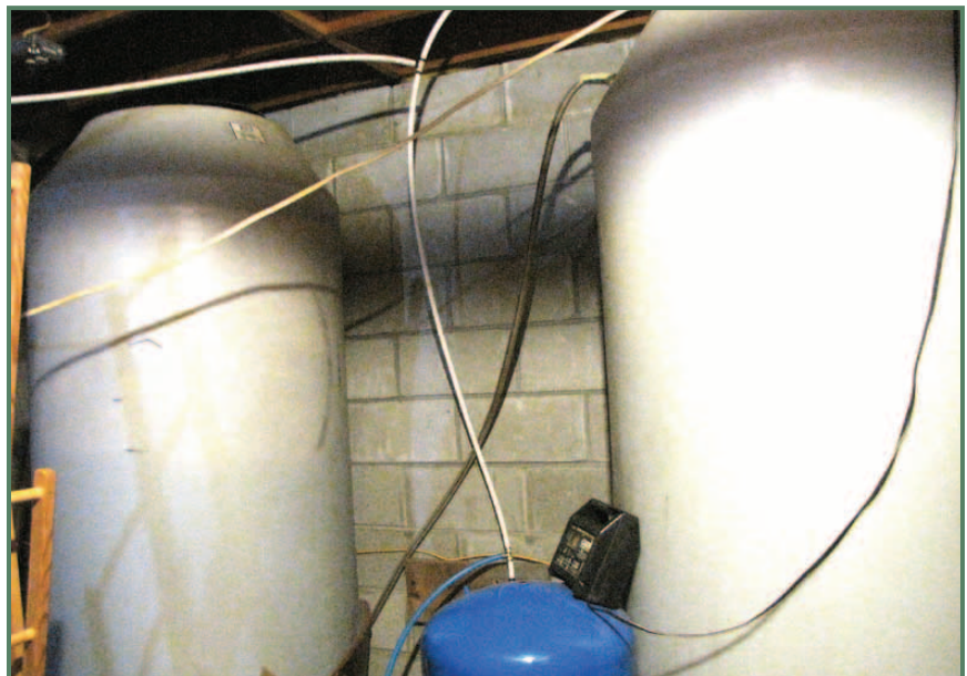
From one 350-gallon tank, we added a second plus a pressure tank to keep the pump from turning on every time we drew water.
