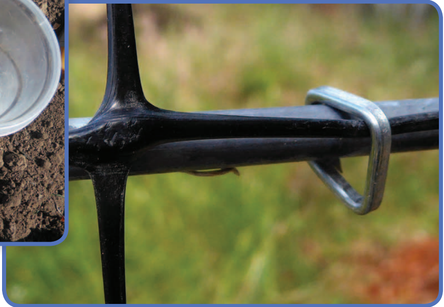
We used hog rings to clip the netting to the cable and to the cattle panels.
