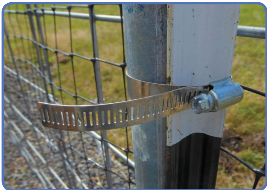
We attached the upright pipes to the T-posts using hose clamps.
